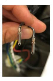
12. Install the newly connected pins from each half of the harness into the two (2) supplied electrical connector shells taped to the wire harness.
