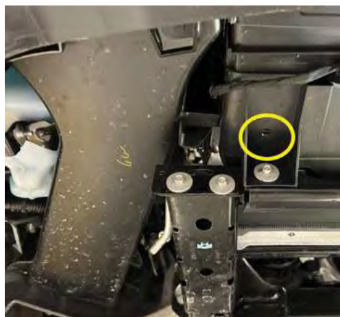
Passenger Side cut hole
